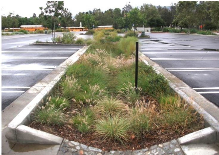
Figure 1151-2: Image of a bioswale within a parking area
