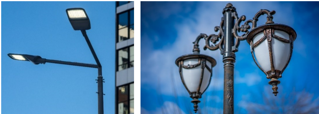
Figure 1154-1: Graphic representations of a full cutoff (left) and non-cutoff (right) lighting fixtures
