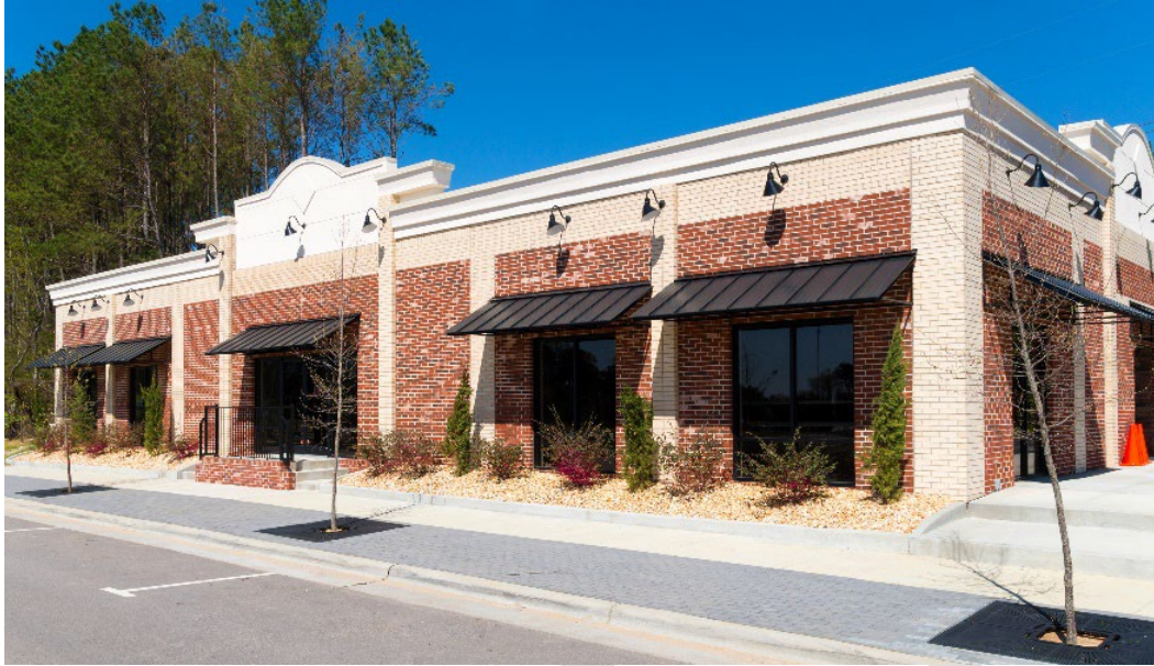
Figure 1132-2: Illustrative example of a building with brick and EIFS accents
