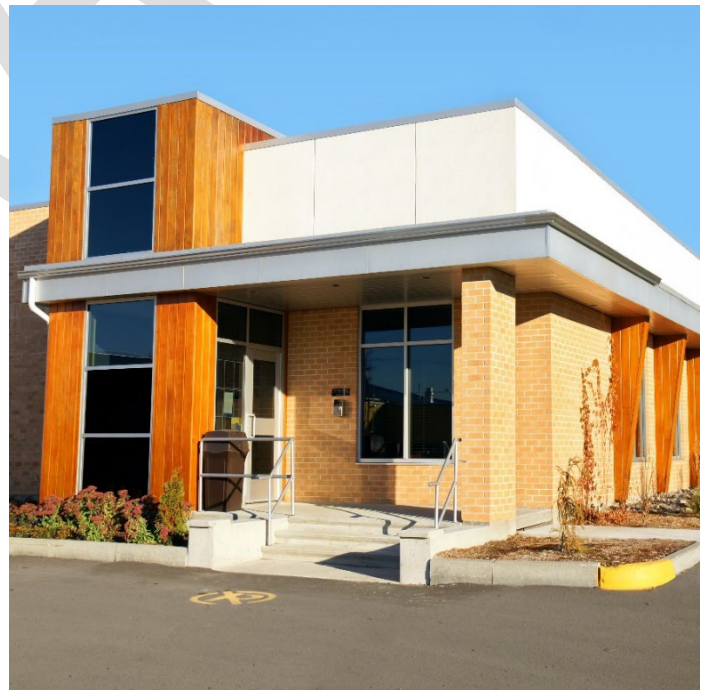
Figure 1132-3: Illustrative example of a facade with different projections, recesses, and material changes
