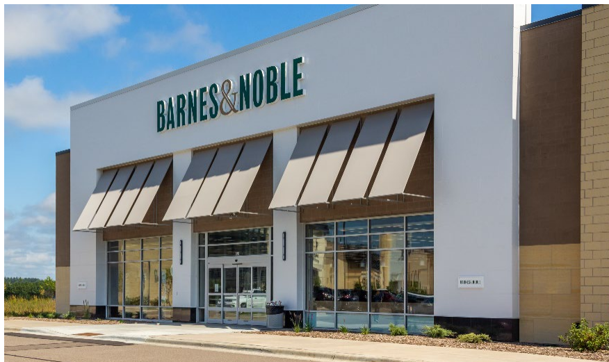
Figure 1132-5: Illustrative example facade with a significant number of windows at the pedestrian level
