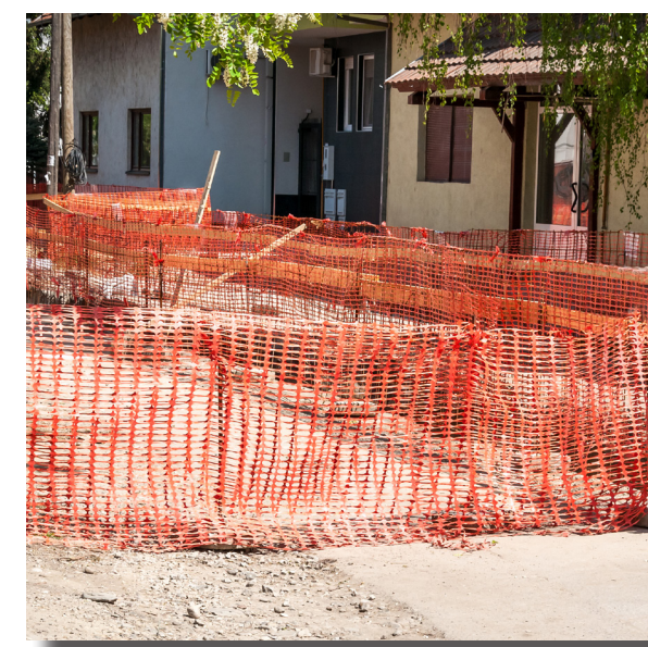
Temporary Construction Material
