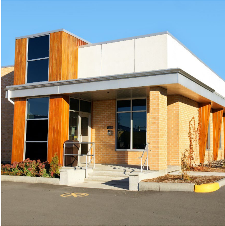
Figure 1133-2: Illustrative example of a façade with different projections, recesses, and material changes
