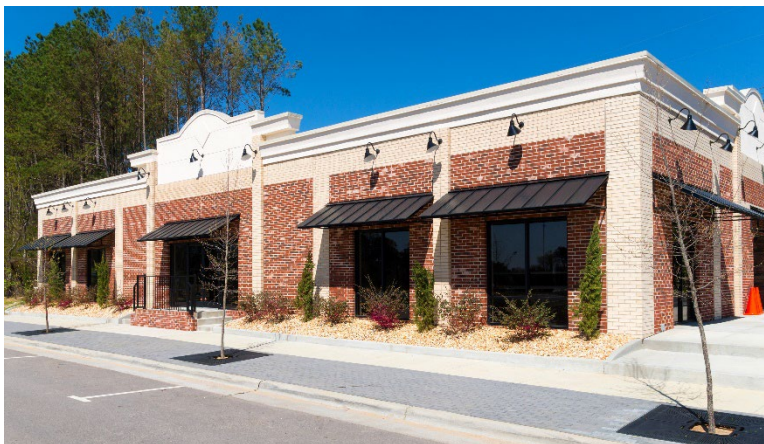
Figure 1133-1: Illustrative example of a building constructed primarily out of brick with EFIS accents
